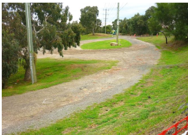
Figure 6: Gravel access road to be re-aligned and sealed
