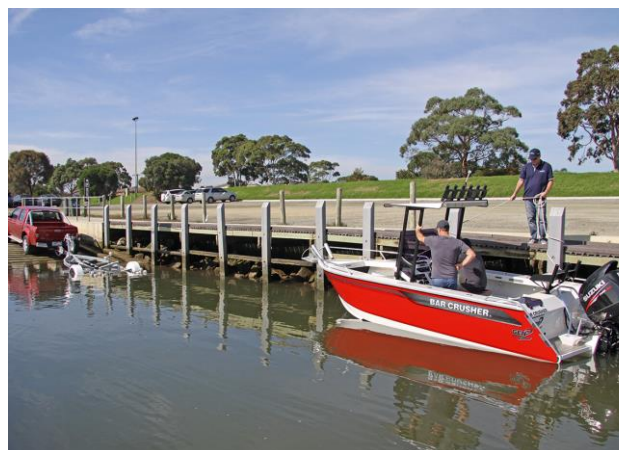
Figure 5: Typical boat holding jetty
